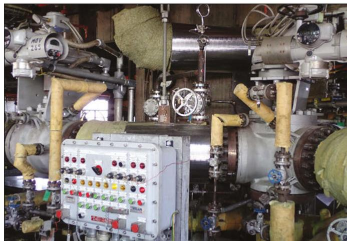
*One of Velan's Severe Service Strategic Business Unit's (SBU) customer-centric offerings this year included three actuated Securaseal metal-seated ball valves, a Programmable Logic Controller (PLC), and local control panels into a single factory-tested package installed in one of the newest delayed coking units in the world.*
