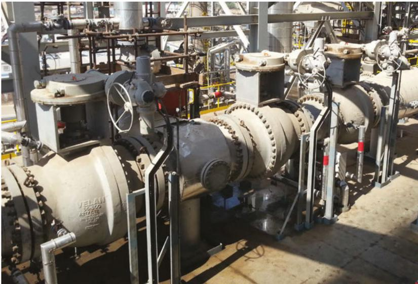
Three 36" Class 300 two-way metal-seated ball valves installed at a refinery in Egypt. Velan's Aftermarket and Technical Services provided on site assistance with the start-up.
