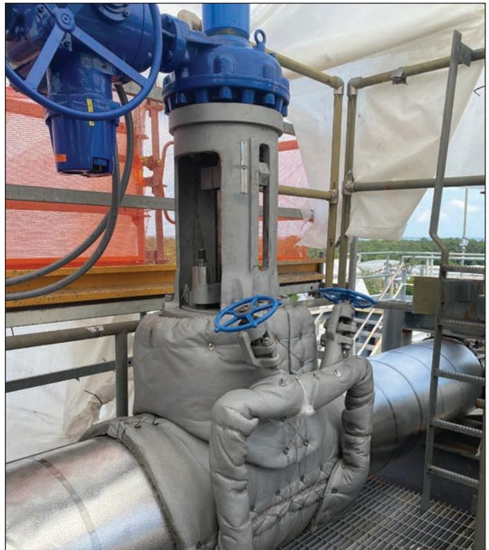
*This 14" Class 2500 forged pressure seal valve, installed in a power plant in Florida—part of a large long-term contract with Velan to supply over 100 (12"–24") valves over 5 years.*
