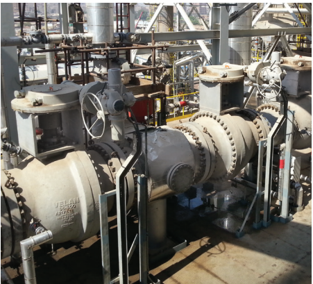
Over 2,600 Velan isolation valves in delayed coker installations
