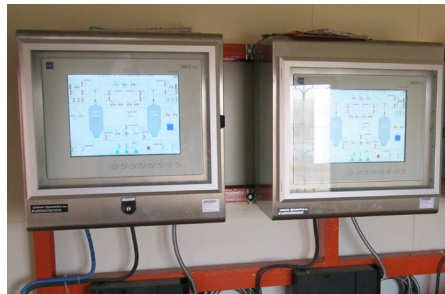
Velan supplied touch screens, to display valve status information for workers in hazardous areas of the refinery.
